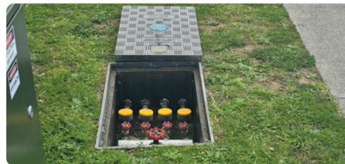
Image - Axioma smart water meters installed
